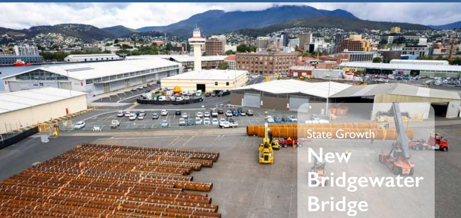
Stockpiles of pile casings for the temporary bridge (left) and permanent bridge (right) located at the Port of Hobart.
