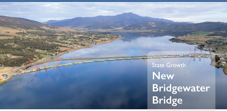
The completion of the temporary bridge, made up of a steel section to the north, and 12 barges to the south, is an important project milestone. This steel platform provides construction access for our workers, plant, equipment and materials across the River Derwent while maintaining traffic flow in both directions on the existing bridge.
