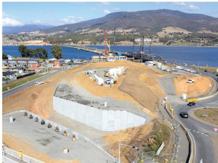
Above, as part of the final design, motorists travelling south from some parts of Bridgewater will access the Midland Highway by driving from Old Main Road into the new Boyer Road underpass. The underpass' reinforced soil slope walls have been completed and will soon have super T concrete beams placed on top. The beams are being produced in Latrobe.
